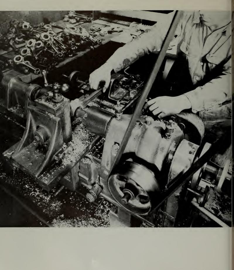
The rod is now placed in a lathe and the babbitt is bored, faced and chamfered. The latter two operations finishes the bearing to standard width.
